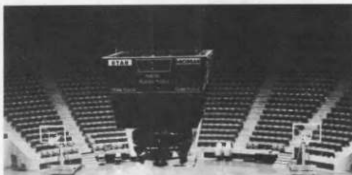
FIG. 13. A typical installation of two-way 500-Hz crossover loudspeaker systems used for sound reinforcement in athletic events and convention centers.
