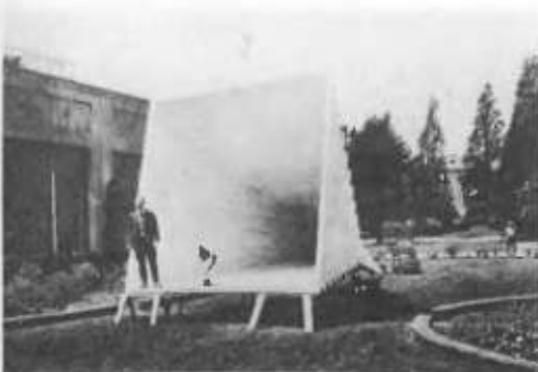
FIG. 2. A moving-coil telephone receiver used as a loudspeaker driver on a very large horn by Pridham in 1915.
